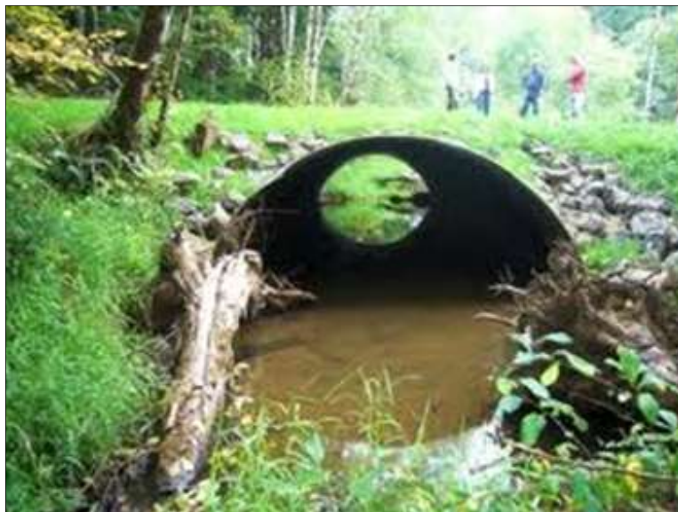
Aluminum box culvert
