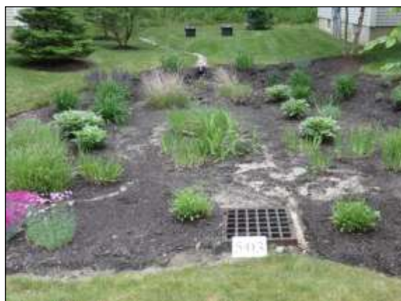
Residential rain garden treats stormwater prior to flowing into a catch basin
